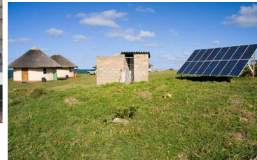
Microgrid for rural settlement
